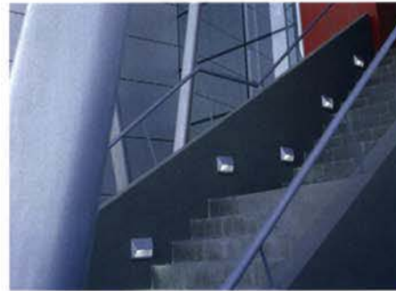
Courtyard lighting - Wall lights
